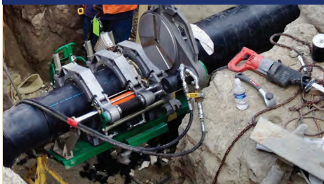
PHOTO 1 HDPE fusion welding equipment in trench.
