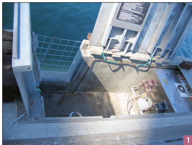
A 6.6-kV connection box on the wharf.
